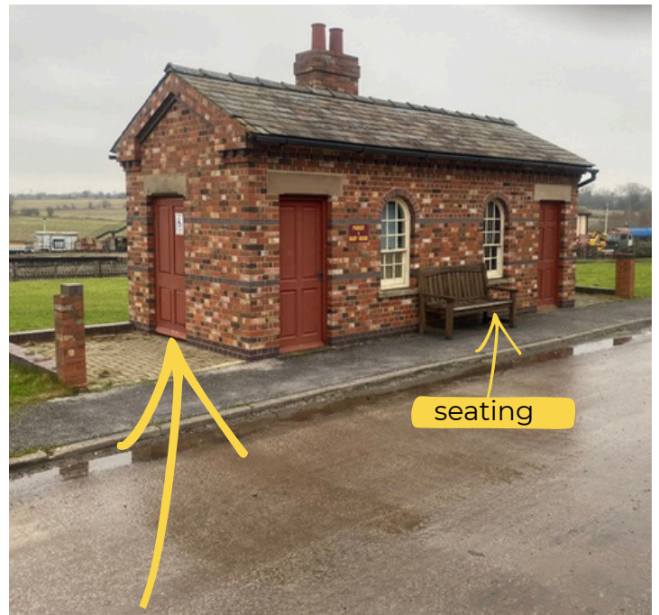
More toilets including disabled and baby change in the centre of Swanwick complex.
